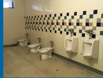
Install Toilet Fixtures in Restrooms at Building 2021
