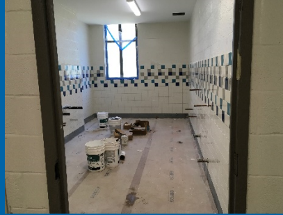
Complete Tile and Epoxy Floors at Building 2010 Restrooms
