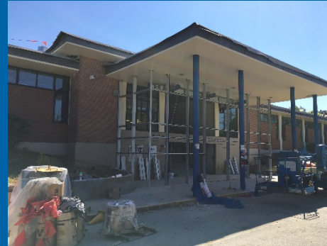
Begin Install of Curtain Wall System at Entry
